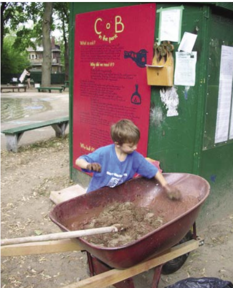
Mixing up dried clay for earthen plaster
